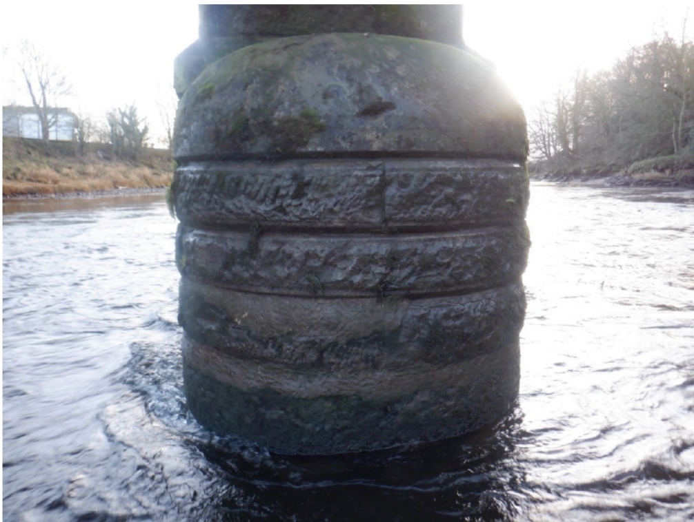
P10 - Pier 3 upstream nose
