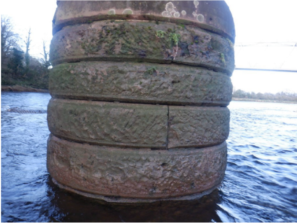
P09 - Pier 3 downstream nose
