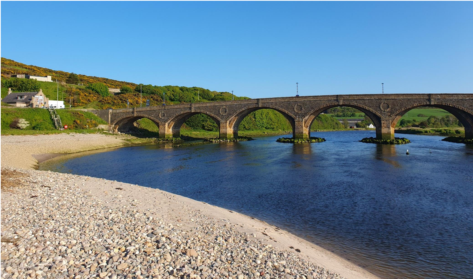
4.1.2 General View of Banff Bridge (taken from the northeast bank, looking south, and upstream)
