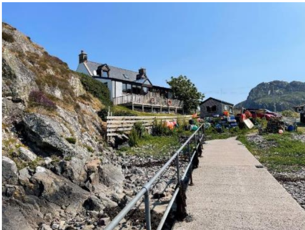
Figure 4. Photograph showing Tarbet jetty, residence/cafe and ferry operating shed with material storage.
