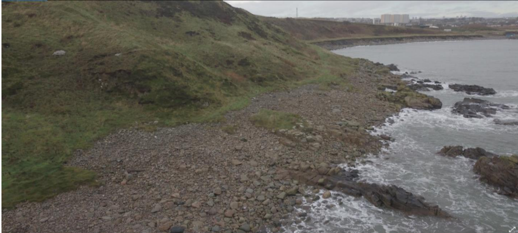
Figure 8: Photographs of East Slope in SSSI taken from drone in December 2018
