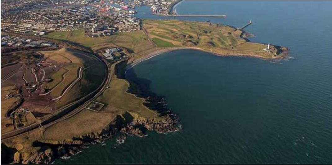
Figure 1.1: Aerial image of Nigg Bay relative to the existing Aberdeen Harbour
