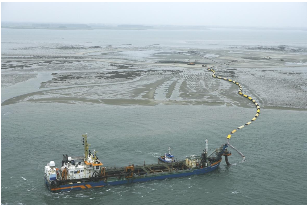
Figure 7.7: Pumping ashore via pipeline system (Van Oord Costa Dorada)
