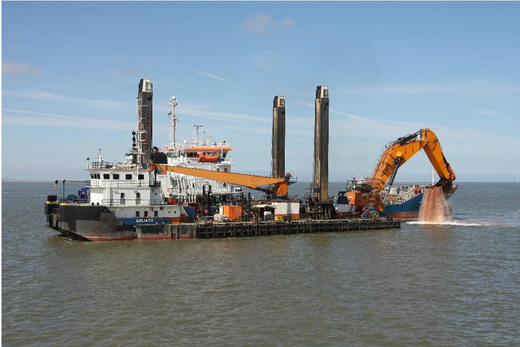
Figure 7.8: Backhoe dredger alongside a Split Hopper Barge (Goliath, Van Oord)
