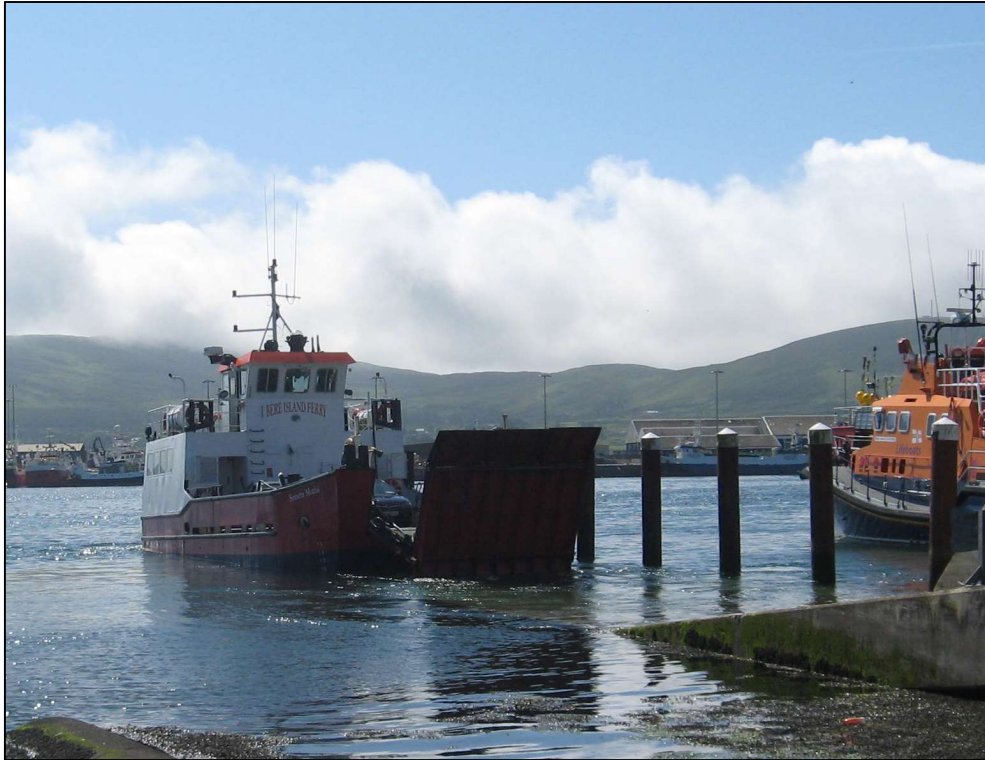
Figure 7-1 Typical Slipway Berthing Piles
