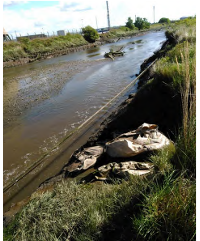
Figure 2: Recent photographs showing deterioration of the site – cable significantly exposed and no longer buried in the river bank
