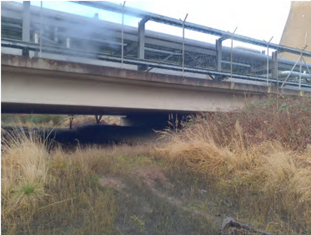
Photograph 4: View of Road 33 Bridge
