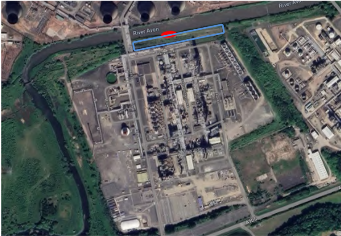
Blue box marking the approximate location of the haul road. The red circle indicating the approximate location of the temporary safeguarding rock bags.
