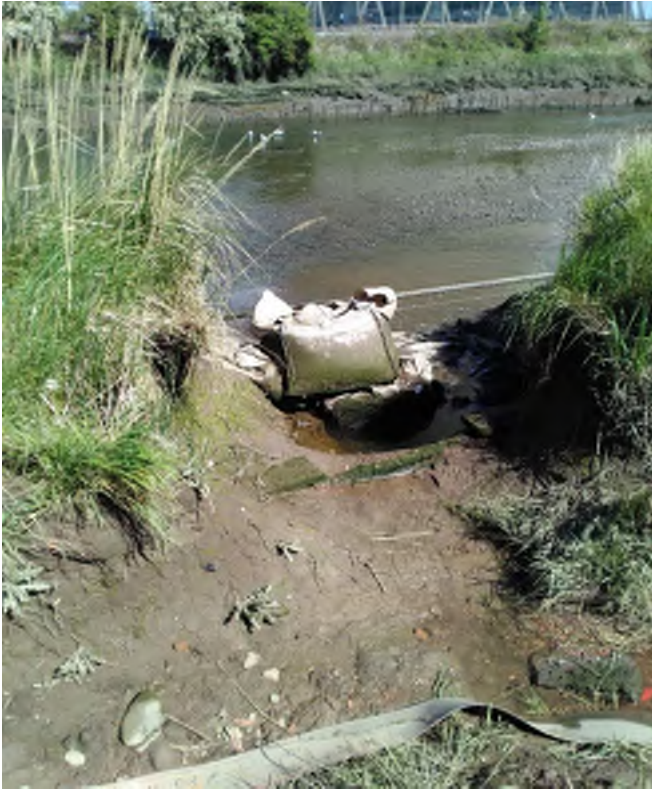
Figure 2: Recent photographs showing deterioration of the site – cable significantly exposed and no longer buried in the river bank
