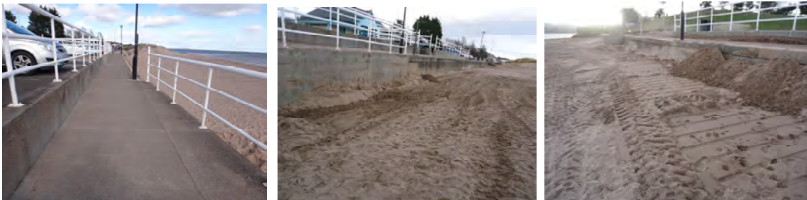
Image 4a, 4b and 4c: Existing River Wall and Upper Beach at Windmill Car Park
