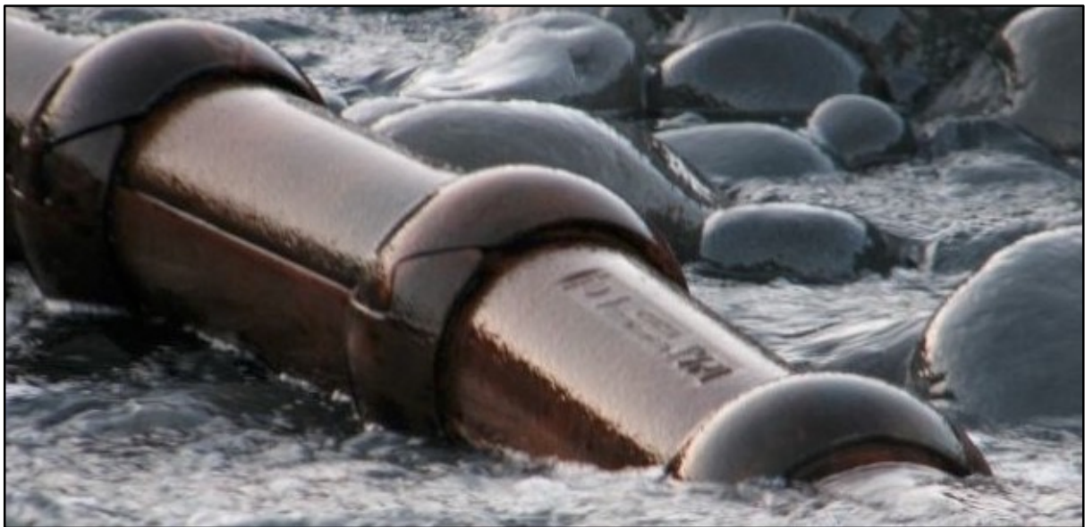
Figure 5 – Steel Submarine Cable Protectors before burial on the foreshore.
