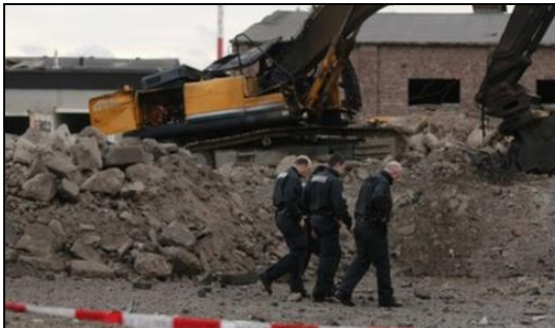
Excavator operator killed by WWII bomb in Euskirchen, Germany – 2014.
