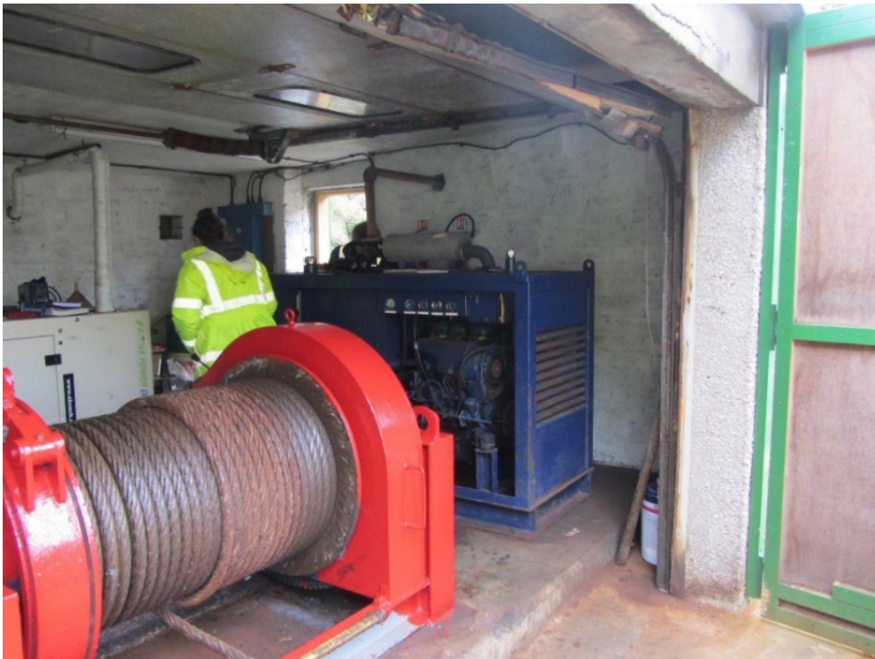
Figure 4-1: The existing winch house on site
