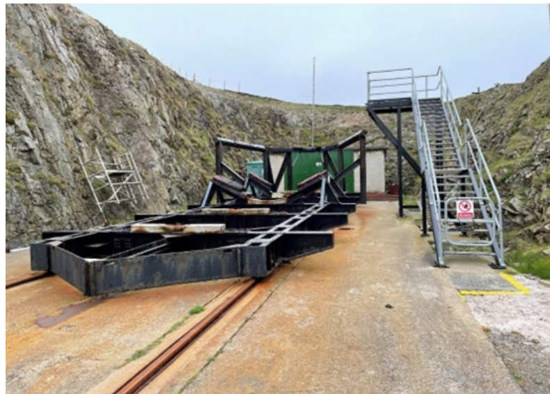
Insert 1: Existing Noust at Fair Isle
