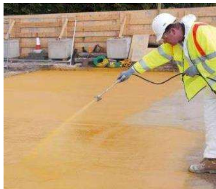
Figure 1.5 – Spray applied waterproofing
