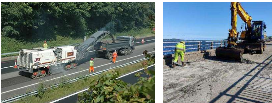
Figure 1.3 – Existing surfacing cold planing & scraping of remaining surfacing
