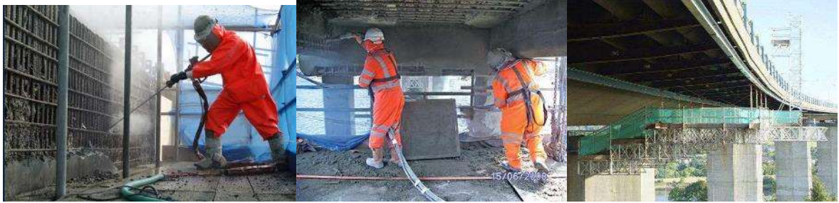
Figure 1.8 – Hydro-demolition, Sprayed Concrete Repair & Access example
