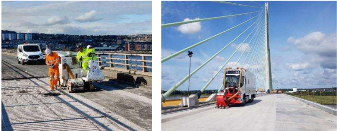
Figure 1.4 – Scabbling of Concrete Deck & Captive Shot Blasting
