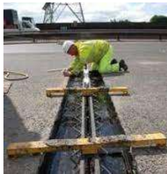
Figure 1.7 – Typical joint installation after new surfacing cut out over gap
