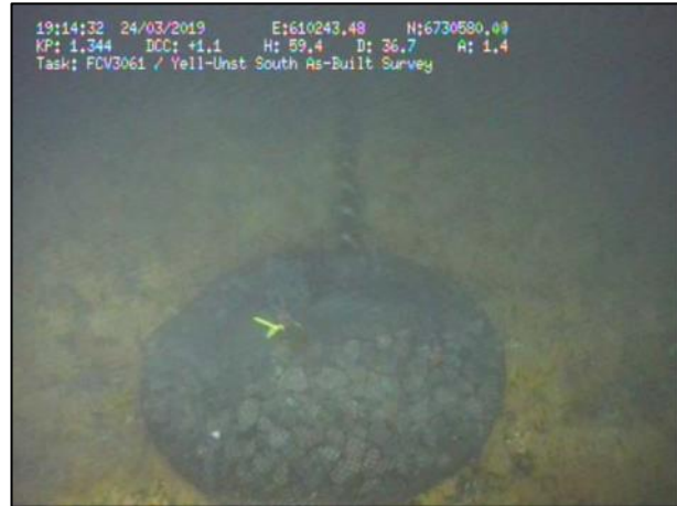
Figure 5-17: Rock Bag in Position Subsea
