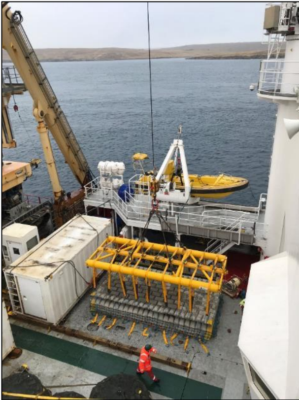
Figure 5-9: Mattress on Deck
