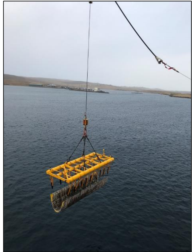
Figure 5-10: Mattress Overboard
