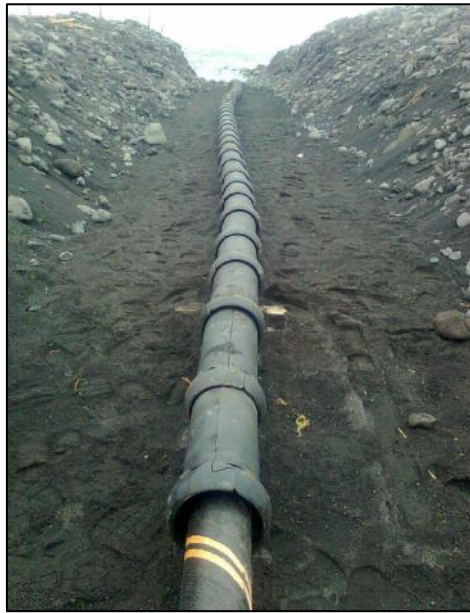
Figure 5-21: Example Split Pipe Installation
