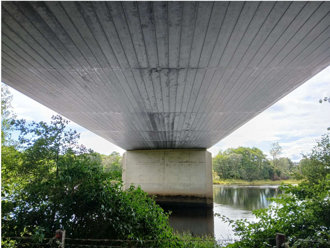
Figure 4. A835 Conon Bridge typical view below the bridge
