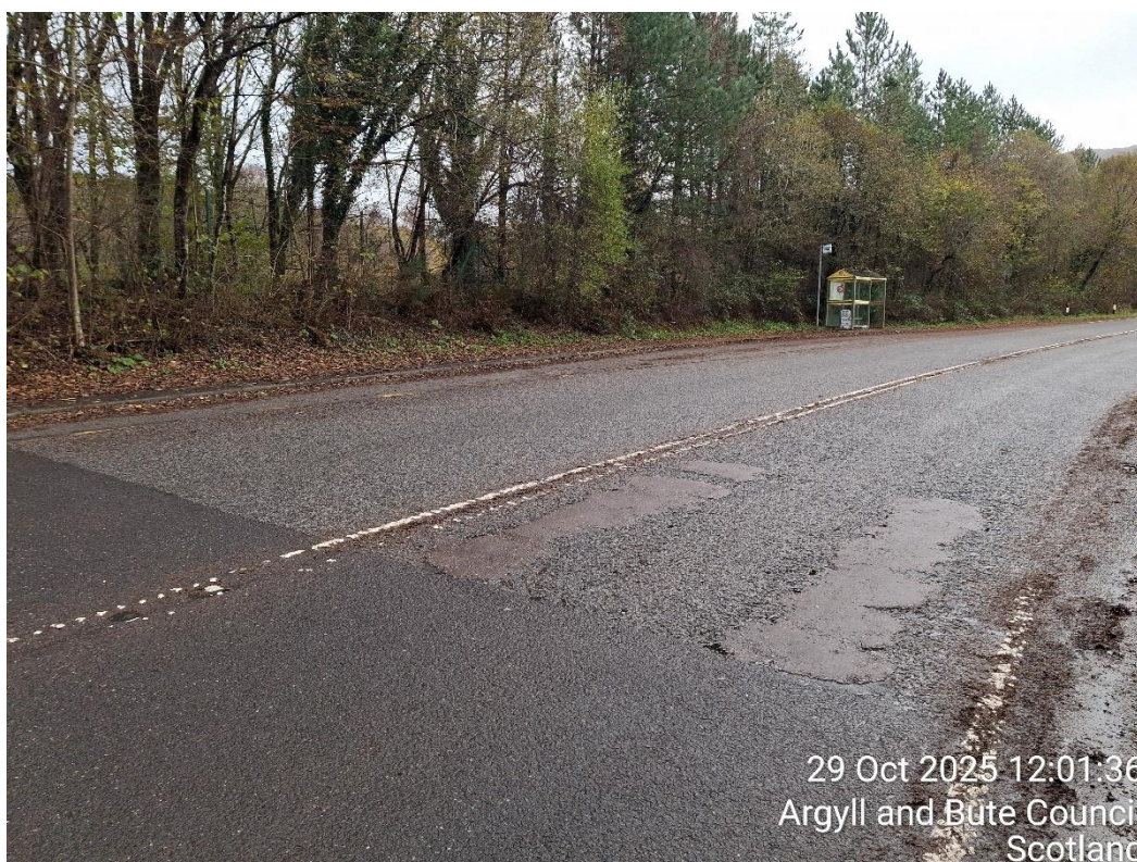
Figure 4: A828 Creagan Bridge southbound view of CL1, showing the end of the scheme extents.
