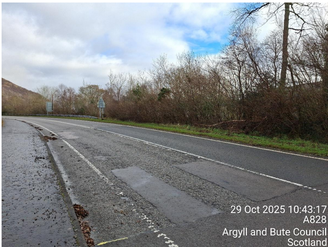
Figure 3: A828 Creagan Bridge northbound view of CL1, showing the start of the scheme extents.
