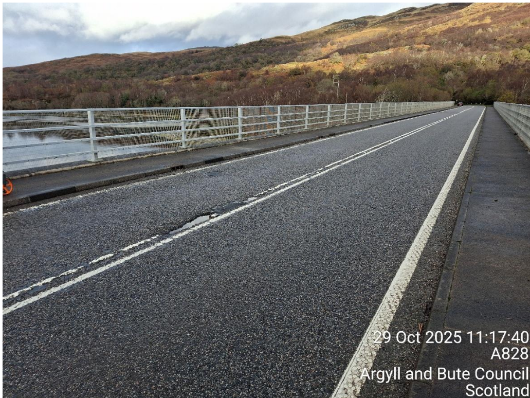
Figure 2: A828 Creagan Bridge typical northbound view above deck.
