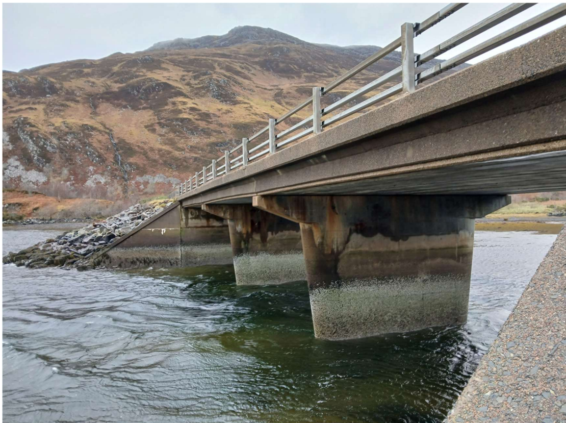
Figure 3. A87 Clachan Duich Bridge typical view below the bridge
