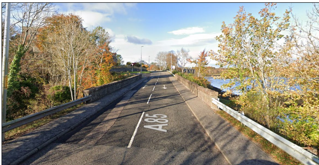
Figure 3: Typical view over the bridge spanning marine environment – looking east to west.
