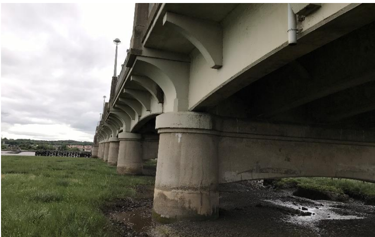
Photograph 2: 50ft Concrete Spans on South Side of the Kincardine Bridge
