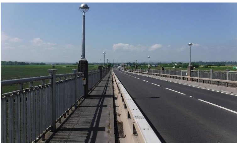
Photograph 3: Existing Varioguard Barriers on the South Side of Kincardine Bridge
