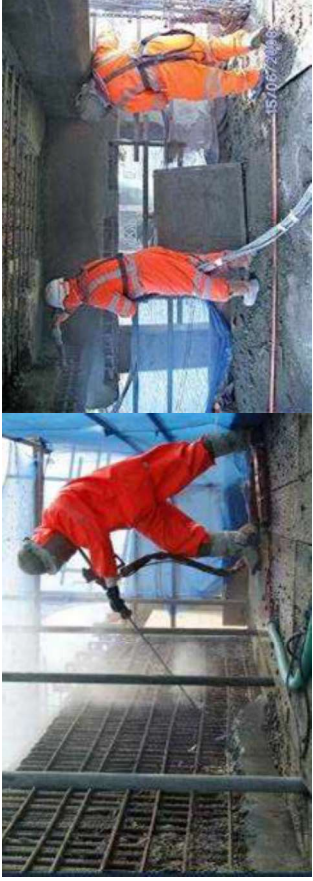
Figure 8 - Hydro-demolition, Sprayed Concrete Repair
