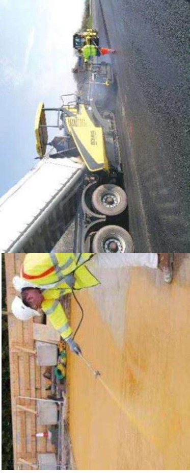
Figure 6 – Spray-applied waterproofing and conventional paving
