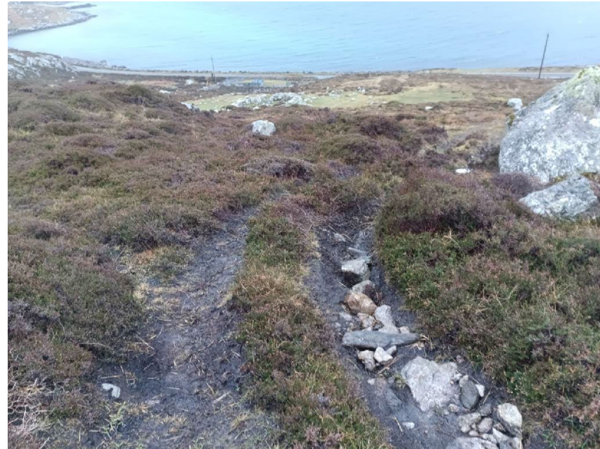
Image 12. Heavily eroded track in the north of the survey area (Appendix 3, Table 8, VE09).
