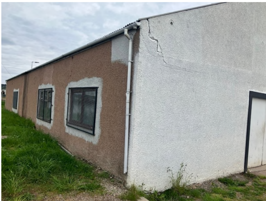
Figure 3.2.1: Boat Shed Due for Demolition
