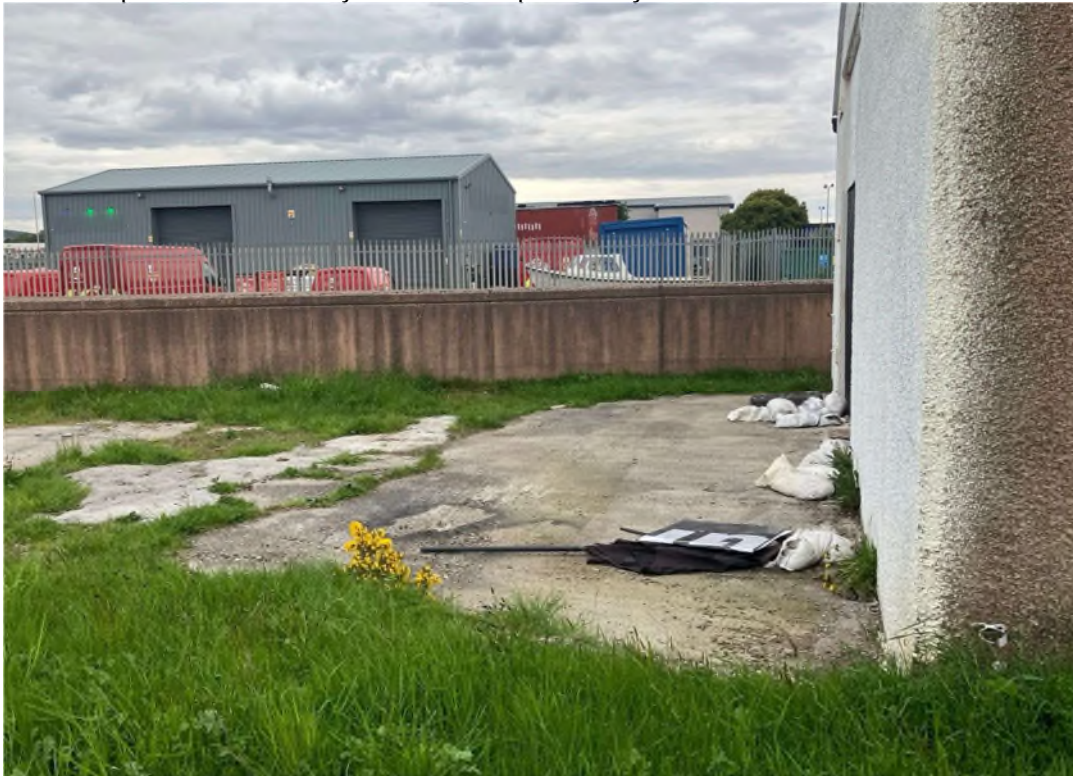
Figure 3.2.2: Hardstanding Behind Boatshed
