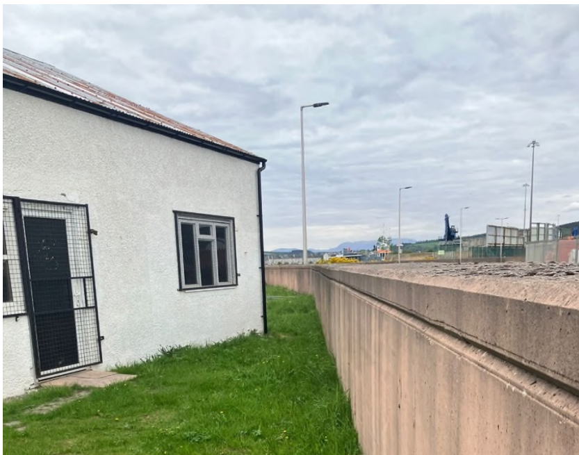
Figure 2.2.1: Boat Shed and Adjacent Flood Defence Wall
