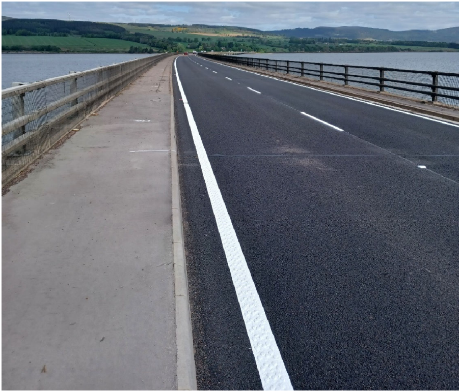
Figure 2, A9 Cromarty Bridge – Typical Northbound View Above Deck
