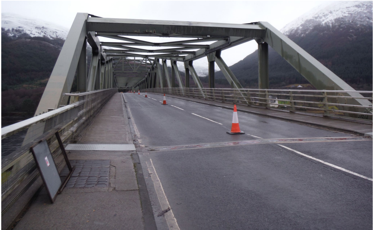
Figure 2, Typical View of Footpaths, Carriageway and Bridge Truss (Facing South)
