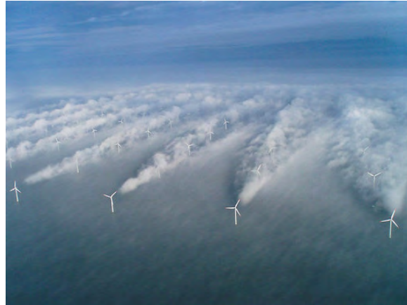
Plate 1: Wind Wake Effect at Horns Rev, February 2008
