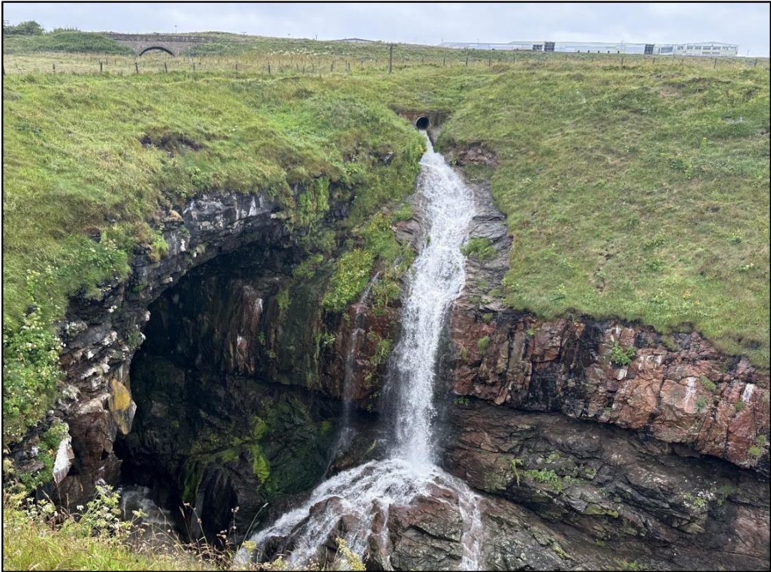
Figure 3-5: Large drainage outlet. Disused kittiwake nests pictured to the left.
