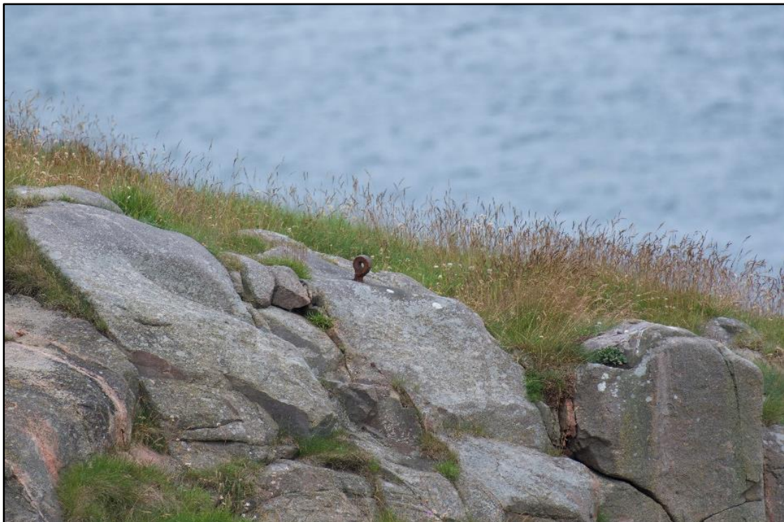
Figure 3-16: Anchor point attached to a boulder at the top of the cliff face. Possibility used for recreational abseiling.
