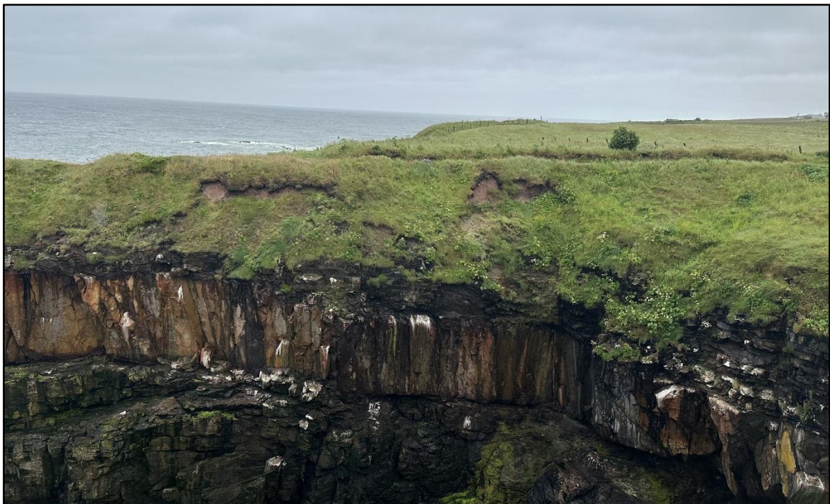
Figure 3-4: Evidence of two small landslides on the embankment above disused kittiwake nests.
