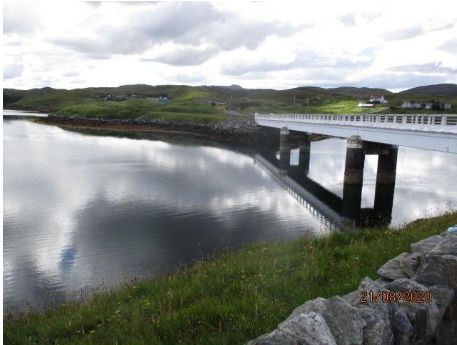
Photo 3.0 East of Existing Looking South
