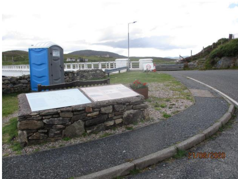
Photo 2.0 North Approach Looking West
