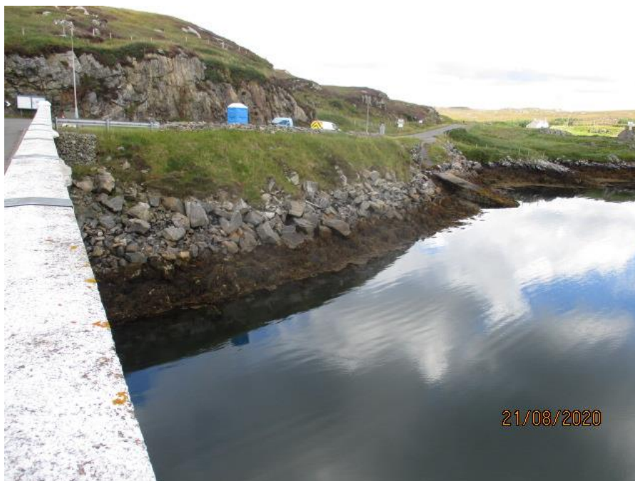
Photo 4.0 East of Existing Looking North
