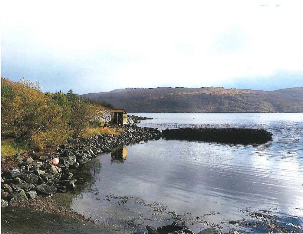
SITE PHOTO from bottom of existing slipway looking south to Loch Sunart.
