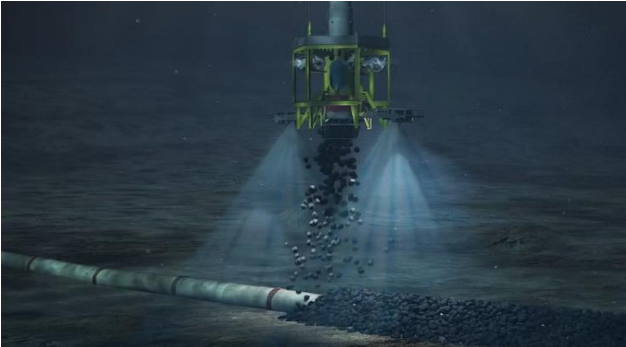
FIGURE 4-8 A REMOTELY OPERATED VEHICLE AT END OF FALL PIPE
