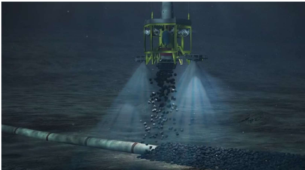
Figure 9: ROV at end of Fall Pipe.
