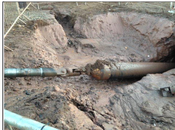
Figure 22. Drilling rod, swivel, pulling head and duct being pulled into the entry pit
