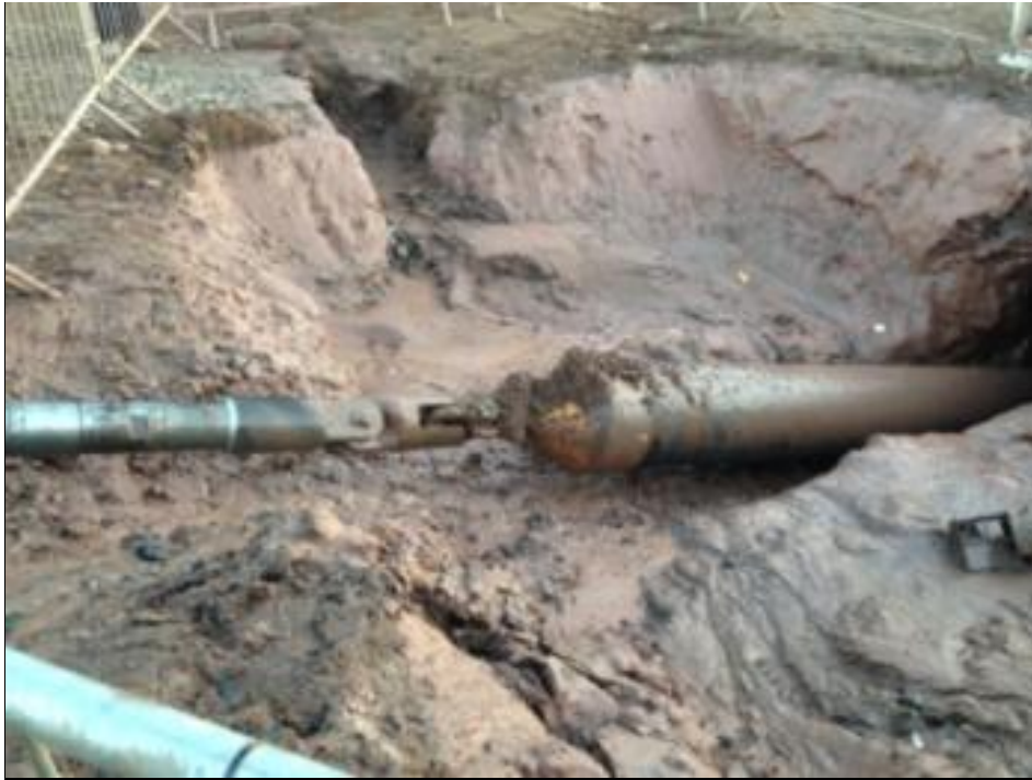
Figure 32. Drilling rod, swivel, pulling head and pipeline being pulled into the entry
