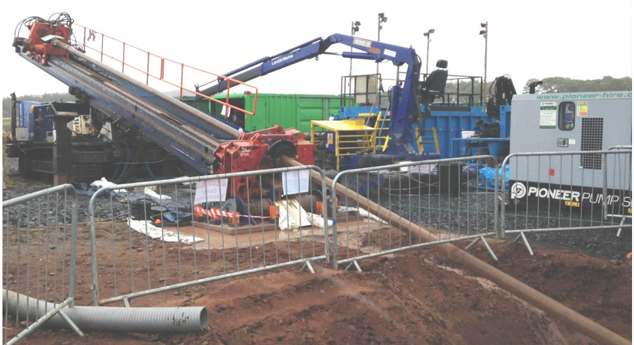
Figure 17. Example HDD rig of the size likely to be used for the HDD's.
