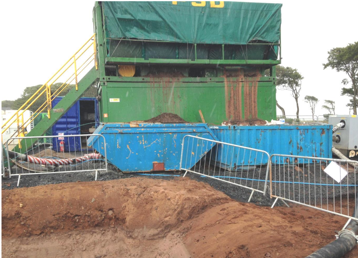
Figure 19. A drilling fluid recycling unit with hydrocyclones and shaker screens on the upper level and active mud tank underneath. The blue bins capturing cuttings as they are removed by the shaker screens. On the right is a grey transfer pump for transferring cuttings from the entry pit (foreground) to the hydrocyclones and shaker screens.
