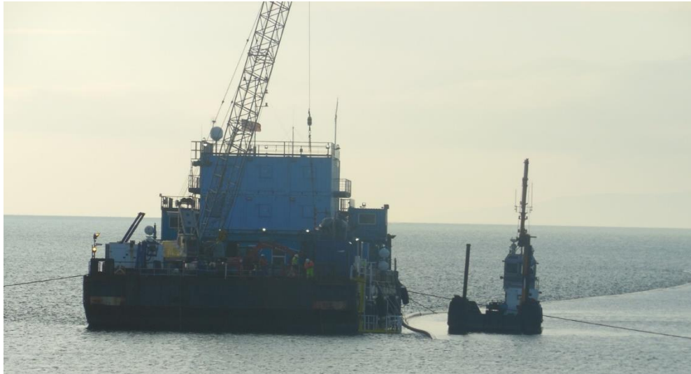
Figure 24. Large barge with four point anchoring and workboat. On the right hand side of the barge the duct can be seen being pulled into the HDD. The water depth is approximately 4m.
