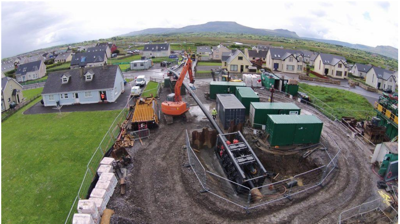
Figure 23. A pipe pusher (black unit at HDD entry point) installing 560mm HDPE on a 584m length HDD in Ireland (AMS Drilling).
