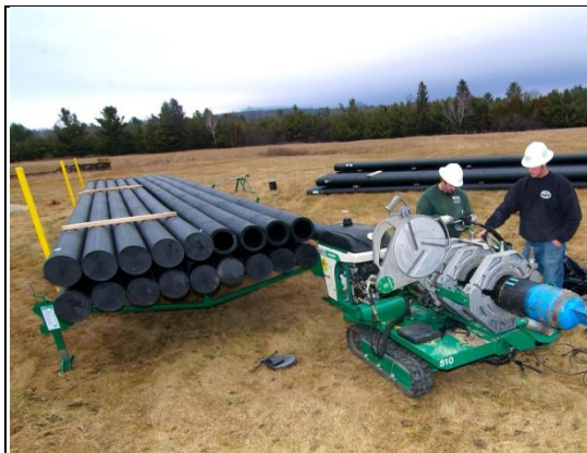
Figure 21. Typical setup of PE butt fusion welder
