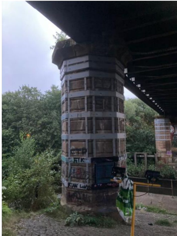
Photograph 1: View of the northern pillar at the northwest side of UB 240/131
