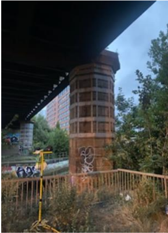
Photograph 4: View of the northern pillar at the southeast side of UB 240/131
