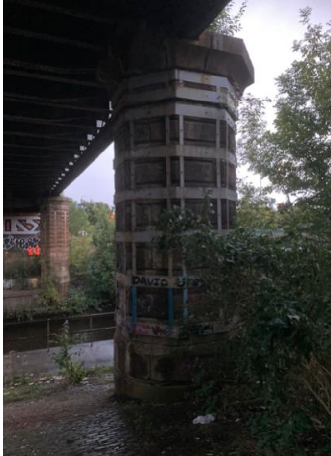
Photograph 2: View of the southern pillar at the northwest side of UB 240/131
