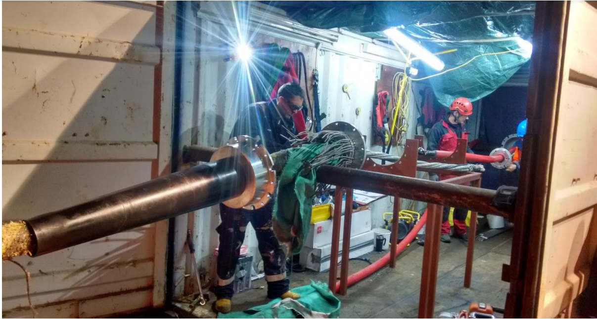
Figure 16. Orbital Marine Power and HV Contractors offshore on a multi-cat vessel cable jointing or “splicing” operations where static cables are permanently connected to the platform cable which supplies power and communications.
