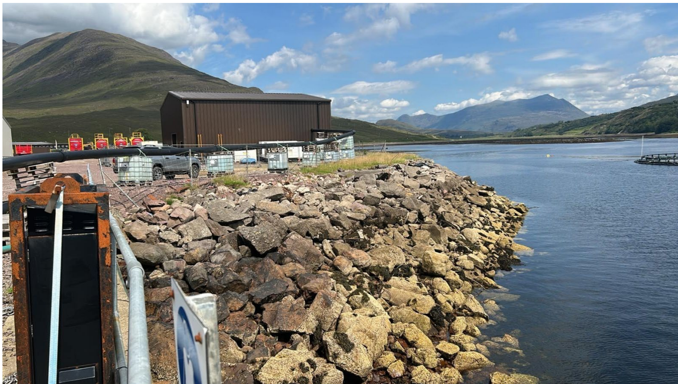
Photograph 3 – View towards where pipe would come ashore, facing NNW.
