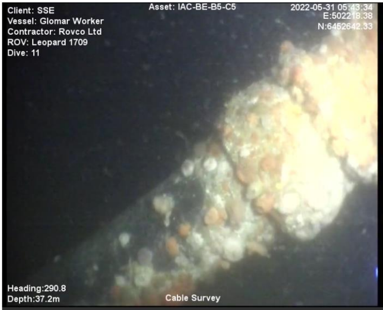
Figure 2.3: Bend-restrictor and bellmouth of J-Tube of IAC-C5-B5 at the C5 end
