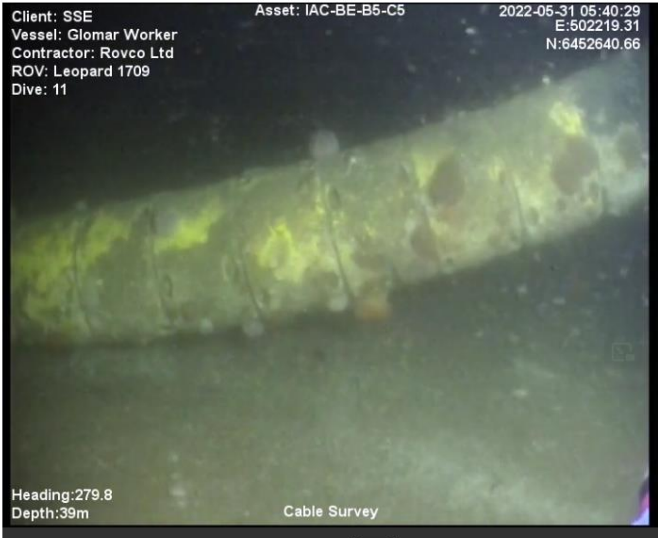
Figure 2.2: Catenary of IAC-C5-B5 at the C5 end
