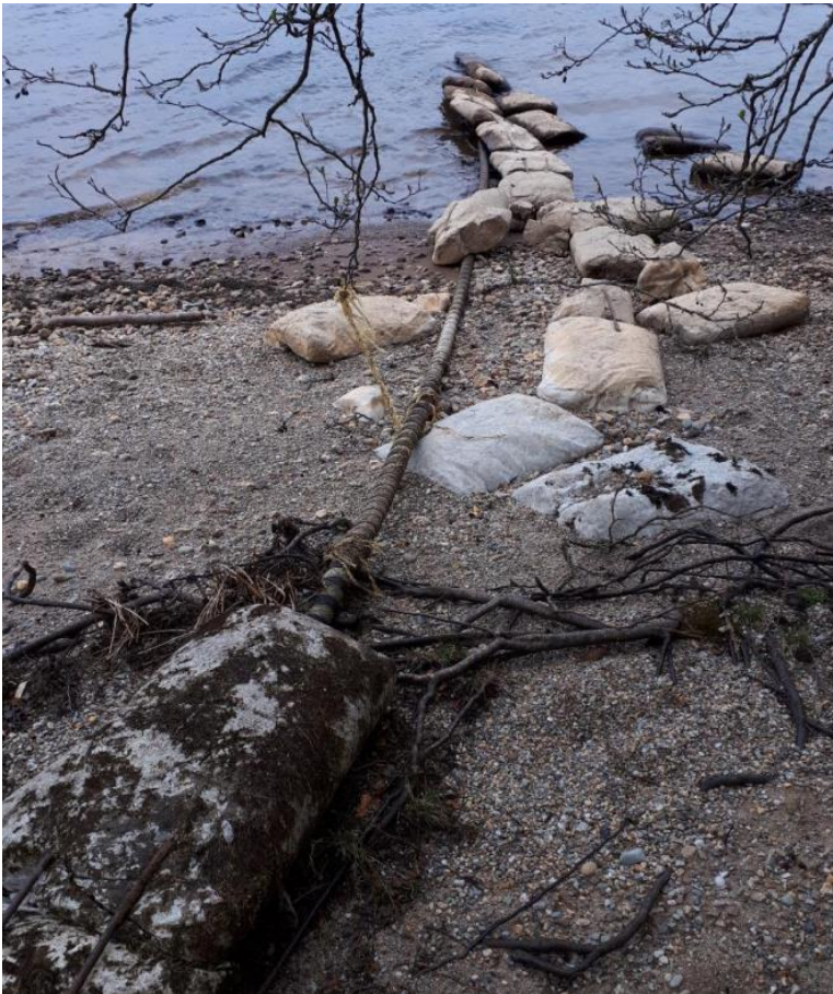
Figure 4- Exposed cable at low water Inchmurrin Island
