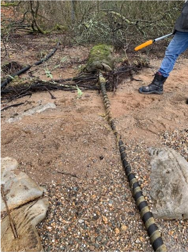
Figure 2 – Exposed cable above MLWS on Carrick Bay
