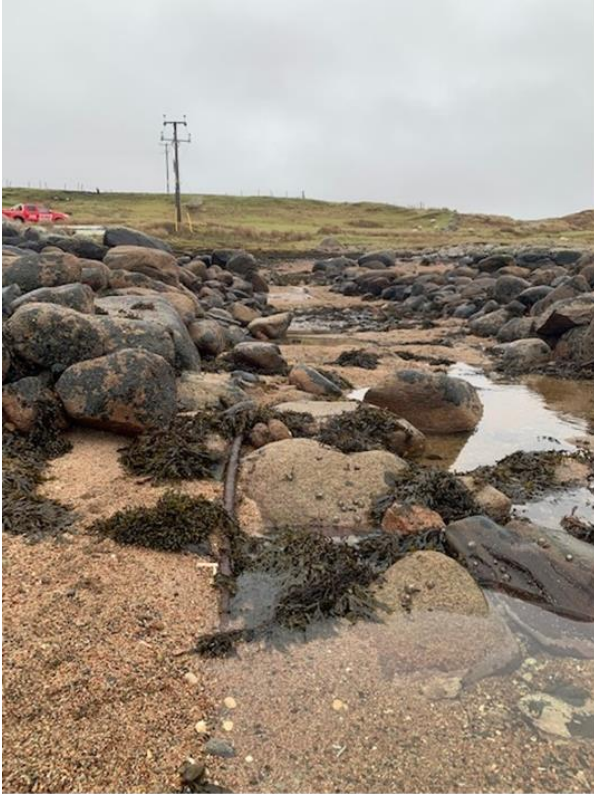
Figure 7 - Mull - Iona (Mull landfall) showing exposed cable
