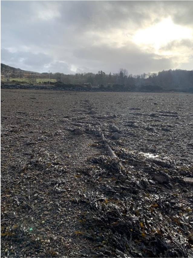
Figure 11 - Overview of cable exposure at Otter Ferry
