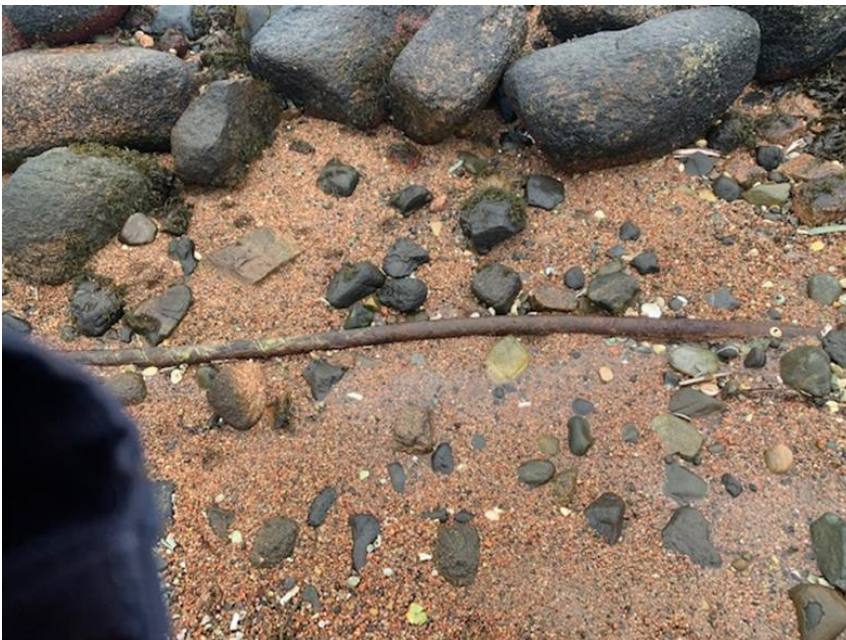
Figure 8 - Exposed cable at Mull landfall (Mull-Iona Island)
