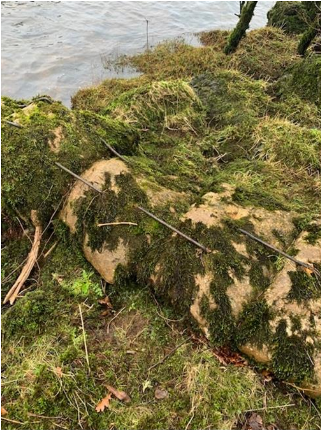
Figure 3- Concrete bags shown at Inchmurrin Island
