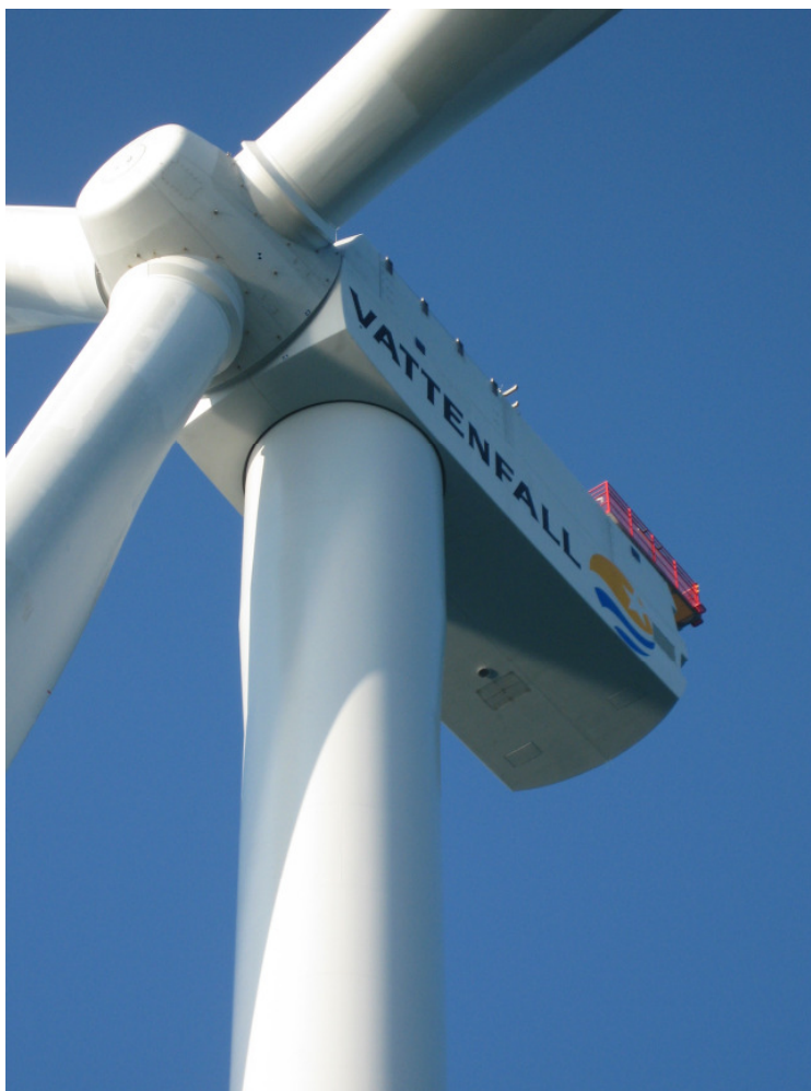
Plate 1.1 A 5 MW Installed Wind Turbine at the Ormonde Offshore Wind Farm
