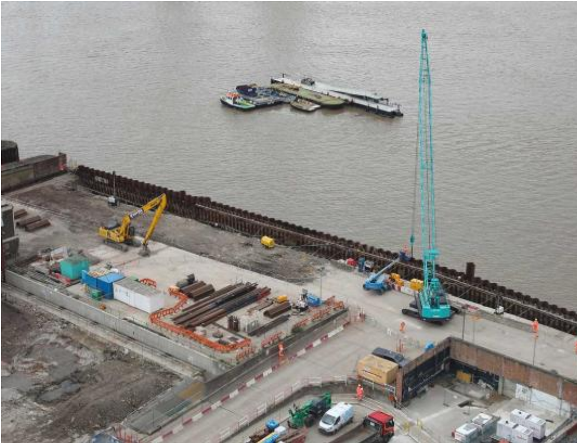
Figure 5 – Typical Crawler Crane
