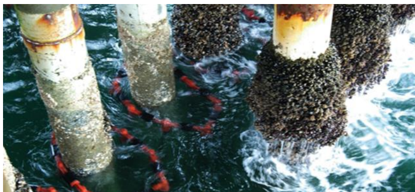
Illustration 4.22: Marine growth prevention solutions (Source: FoundOcean Ltd)
