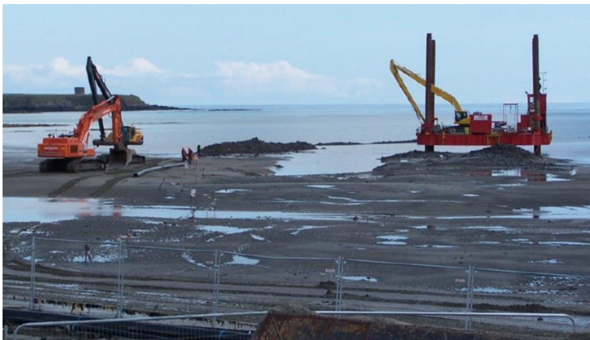
Illustration 4.20: Open cut trenching beach excavations – tracked excavators and barge-mounted excavators (Source ETA Ltd)
