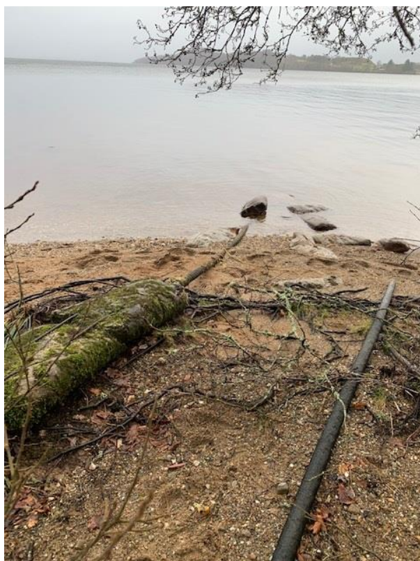
Figure 1 – Remedial work required at Carrick Bay
