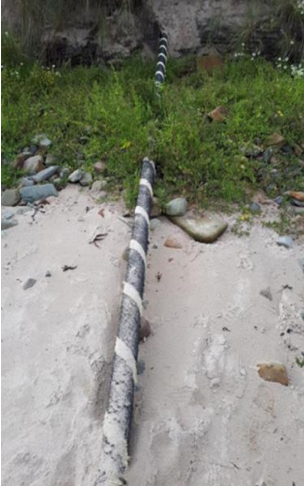
Figure 16 - OOS Cable on Eday entering the Sand dunes
