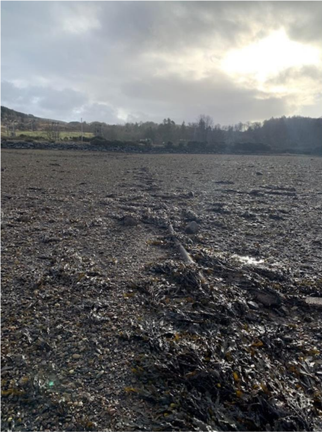
Figure 11 - Overview of cable exposure at Otter Ferry
