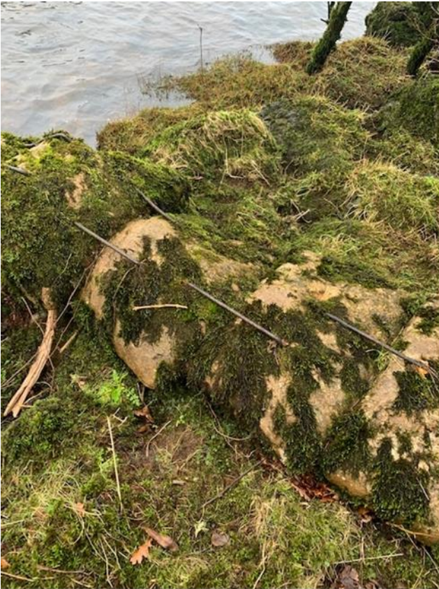
Figure 3- Concrete bags shown at Inchmurrin Island
