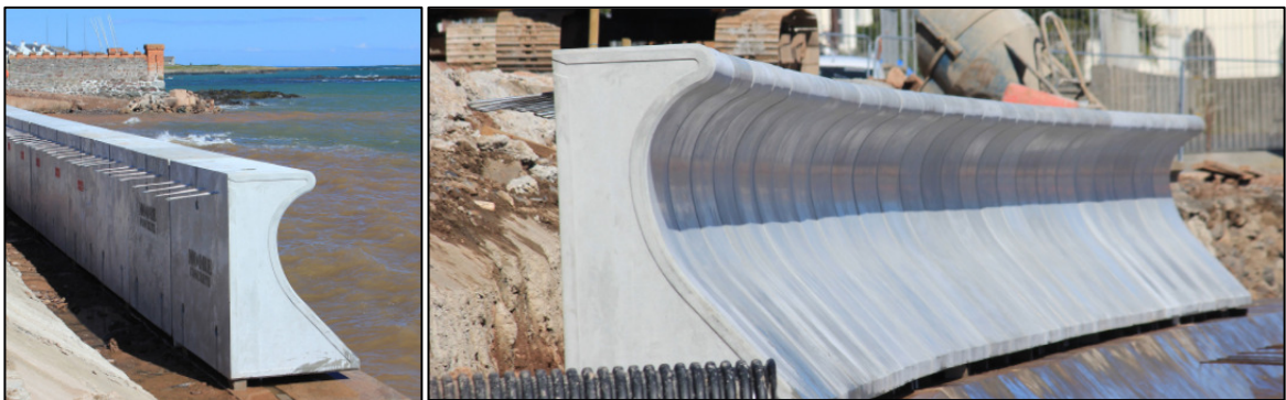
Figure 1 and 2: Examples of proposed precast seawall
