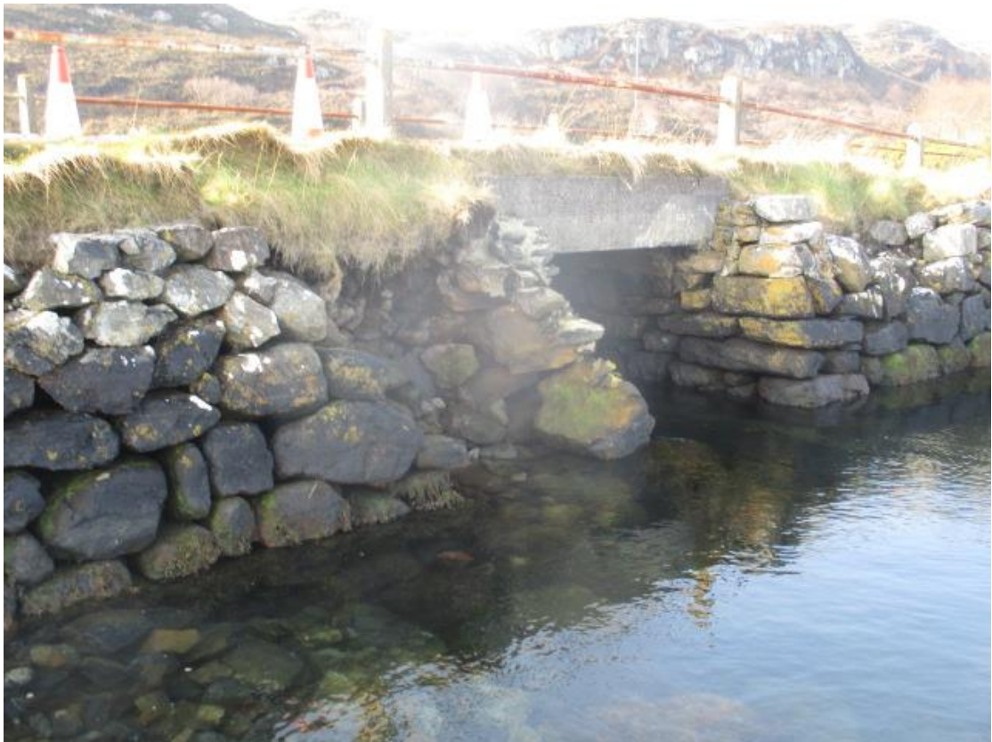
Collapsed wall section adjacent to bridge opening
