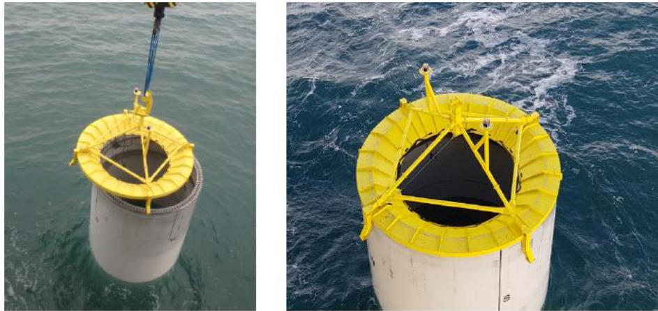
Figure 4-9: Example of a monopile cover installation.
