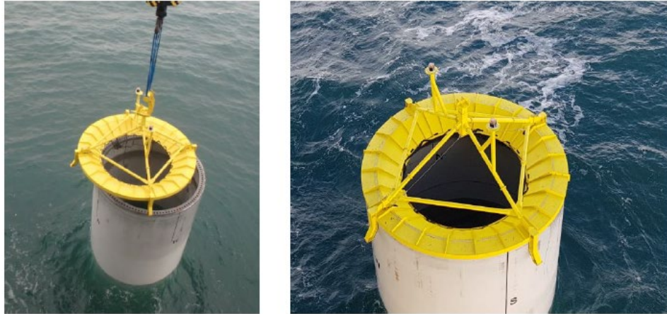
Figure 4-9: Example of a monopile cover installation.
