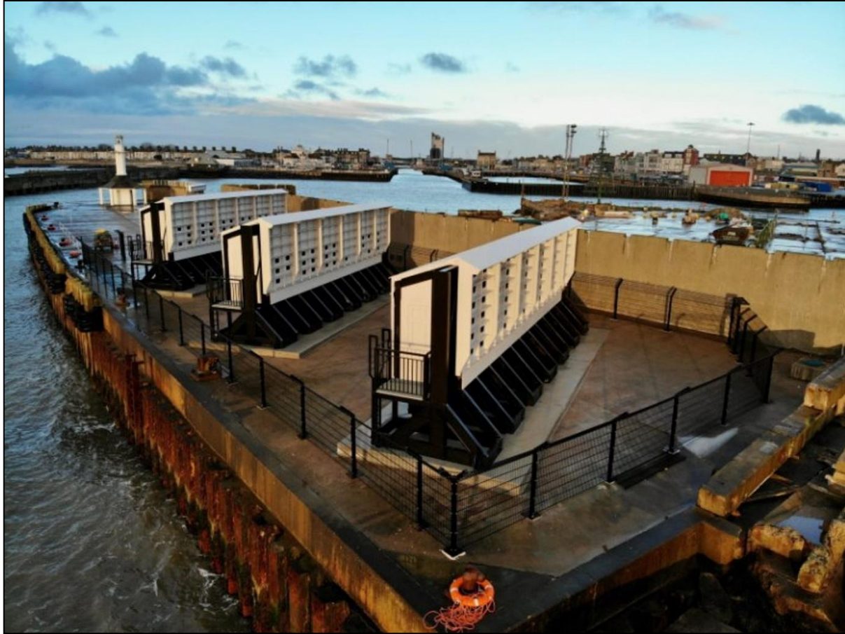
Figure 2: Onshore kittiwake nesting structure constructed for the East Anglia and Norfolk compensation (Vattenfall, 2023) 3
