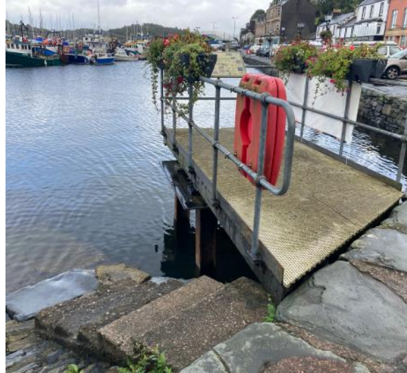
Fig 2.3.2 Existing historic slipway & viewing platform @ John Renshaw Architects
