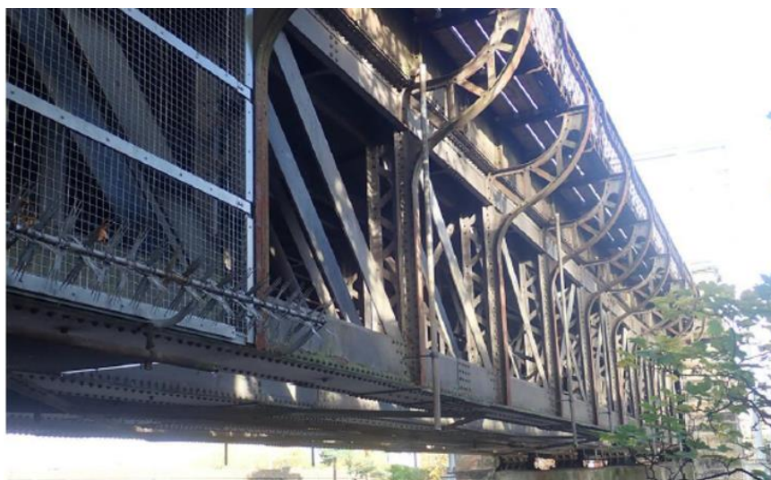
Figure 5-External Drainage pipe installed vertically along the main girders
