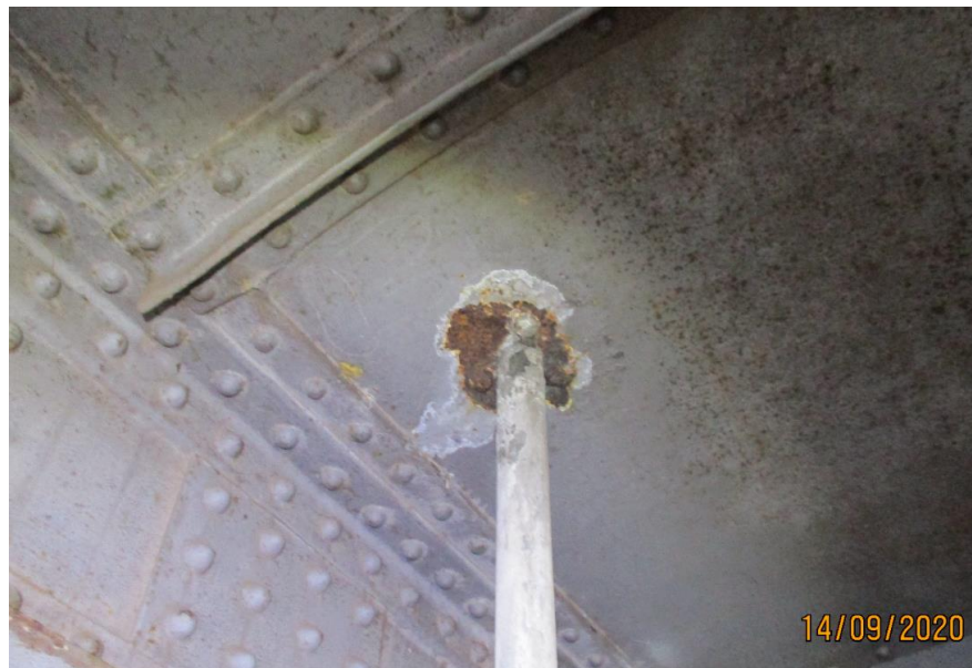
Figure 7- Radial corrosion to buckled deck plate around the drainage pipe
