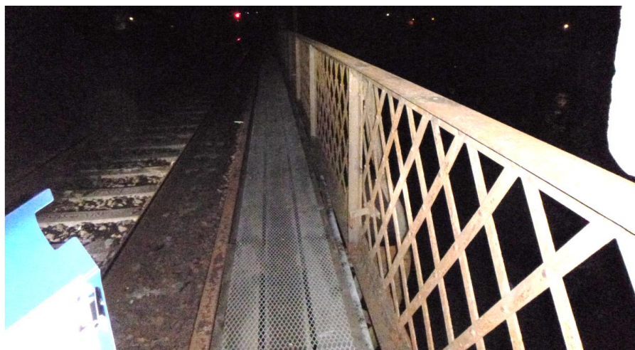
Figure 9-Trackside walkway, comprising longitudinal timber and grid mesh panel spanning along parapet girders (DK2-4)
