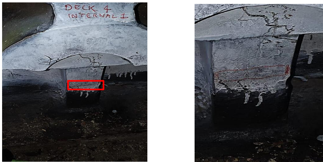
Figure 4-1 No. Crack to the outstand of the bearing extracted from LWC-Forth Viaduct 014
