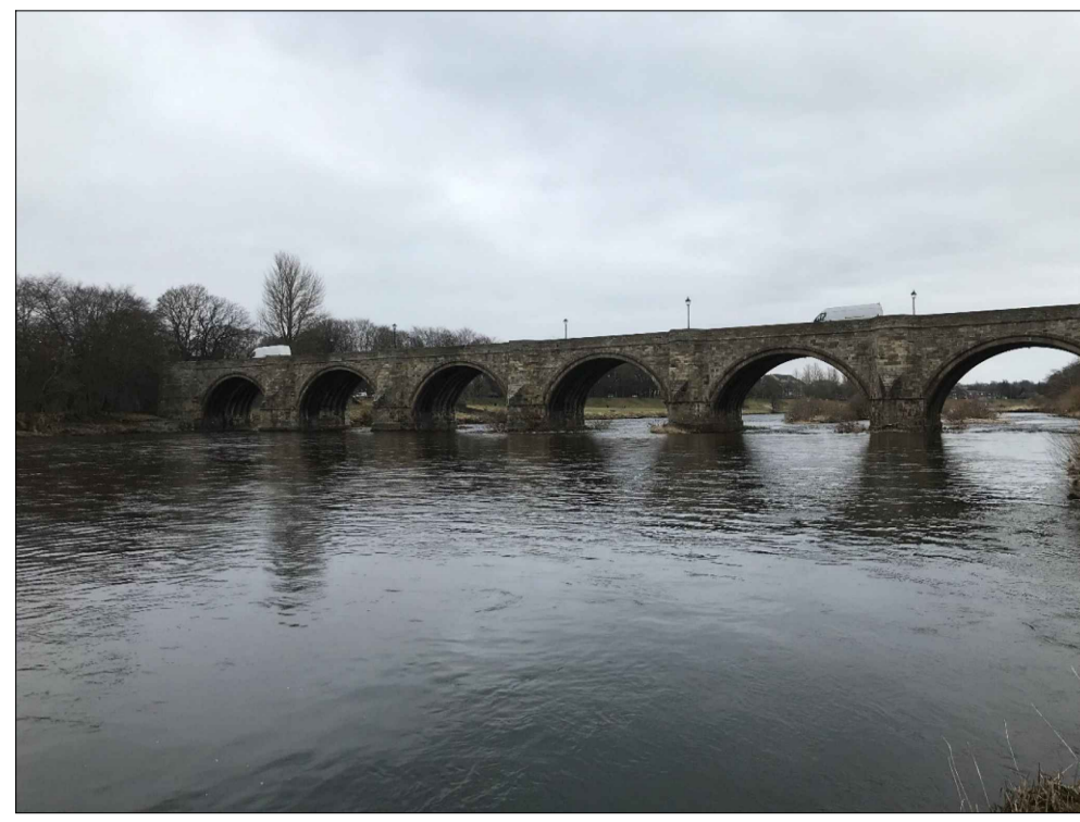
PHOTO 1 - DOWNSTREAM VIEW TO THE BRIDGE SCALE 1:25
