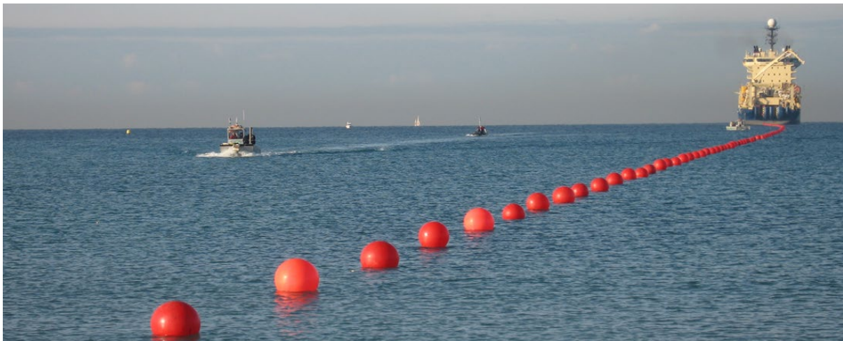
Cable Pull in Progress Rates – 1 day per landfall
