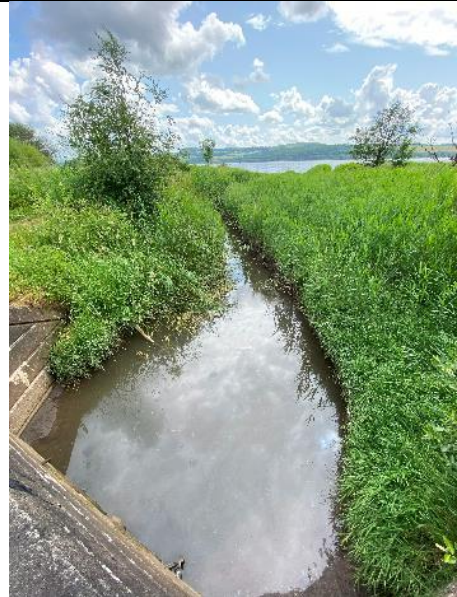
Plate 10: Hunter's Burn's current culvert outflow and confluence with the River Clyde.
